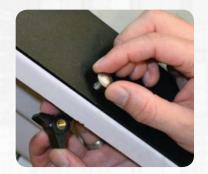
Remove the six flat bars by unscrewing the tri-knobs underneath and removing the pass-thru bolts.
