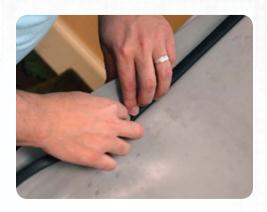
Pull out the barrier retaining ring and then remove the barrier.
