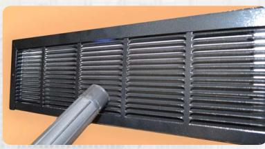
If your Hydromassage Lounge uses an external cooling unit, examine the intake fins on the cooling unit. If any dust build up is present, merely vacuum the intake side.
