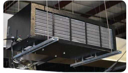
CEILING MOUNTED TEMPERATURE CONTROL UNIT
