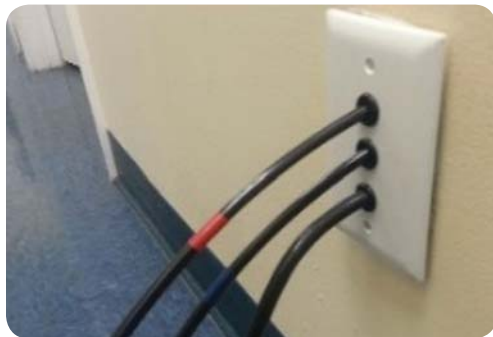
RUN WATER AND POWER THROUGH WALL CONDUIT WHERE POSSIBLE
